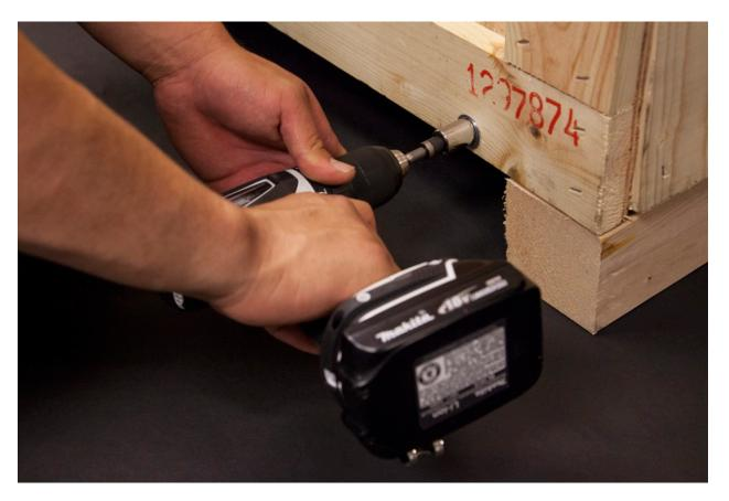
2. Using a 9/16" socket bit attached to a cordless drill or socket wrench remove the 10 bolts around the bottom of the crate.
